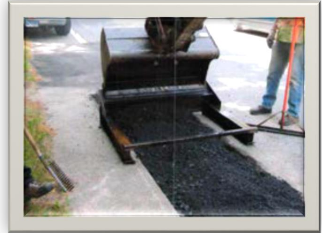
Asphalt Trench Paving Box
