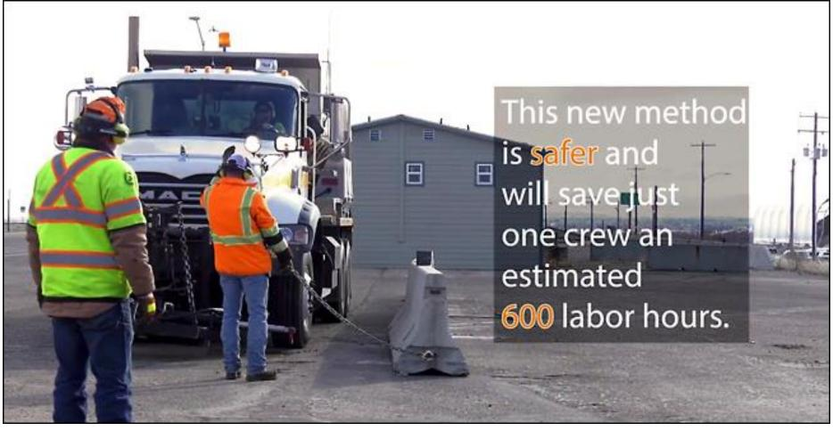
The maintenance crew in Caldwell has a perennial job of realigning jersey barriers that are hit by cars. It takes them days to cover the miles of barriers within the urban Interstate 84 corridor. The crew machined a hydraulic attachment for a plow truck that is much safer and faster than the old method.
