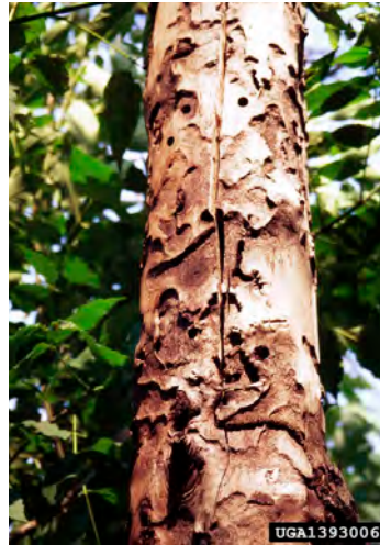
Damage under bark
