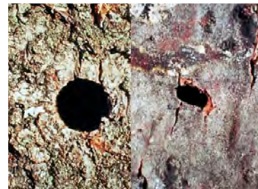
Two types of wood borer exit holes
