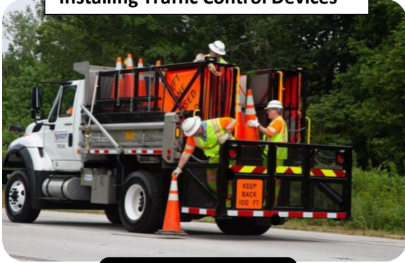
Installing Traffic Control Devices
